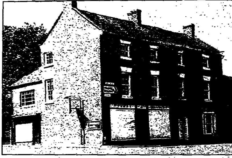
Walford House, Drayton Road, Hodnet, Shropshire. The early three-story 19th-century brick house has a plain tile roof, four sash windows on the first and second floors, a double shopfront on the ground floor.
